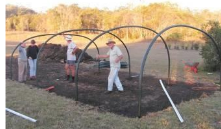
Top: ceiling batten. L to R: poly-pipe arch; star picket; shade-cloth with tie-wires on it; timber upright. Not on photo: door; hinges; latch; metal strapping and tacks; brackets, threshold, weed mat.
